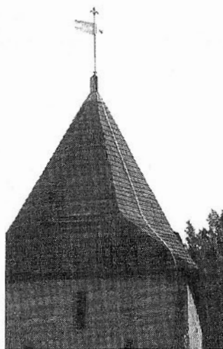
Fig. 1: Lightning arrester on church spire.
